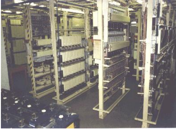
Photo of a working Strowger exchange at Catford, UK. Photo by Martin Loach https://commons.wikimedia.org/wiki/File:Catford_Strowger_Switch.gif
